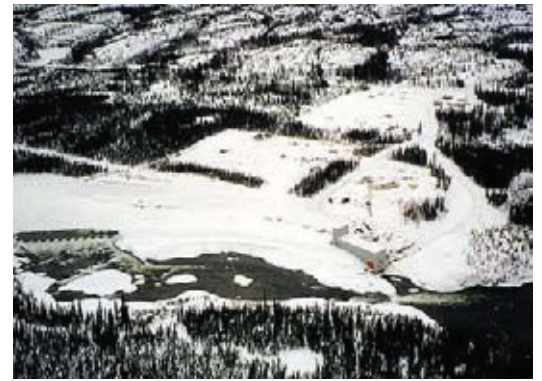
FIGURE 4 Snare Cascades hydro power plant, the latest addition to the Snare Hydro facilities in 1996. / La centrale de Snare Cascades, dernière addition terminée en 1996.
